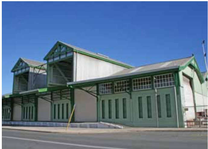
B shed has been externally painted in its original colours.
