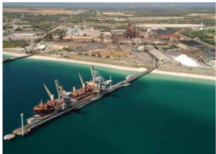
Kwinana Bulk Berth 2 at Fremantle Ports' Kwinana Bulk Terminal.
