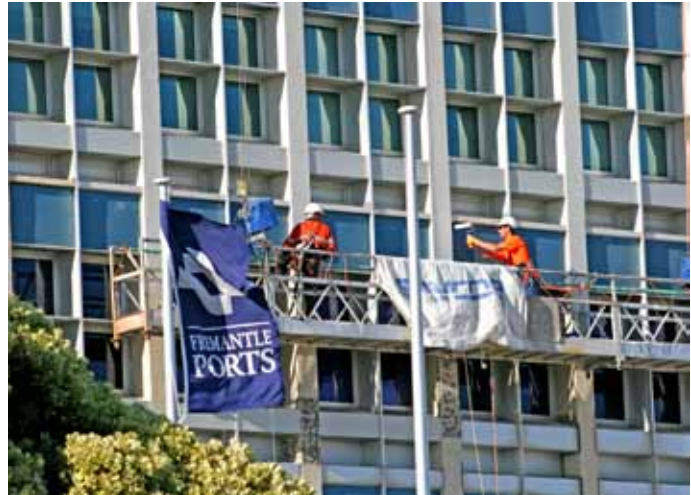
Administration Building repairs have been necessary to counter the impacts of weathering.
