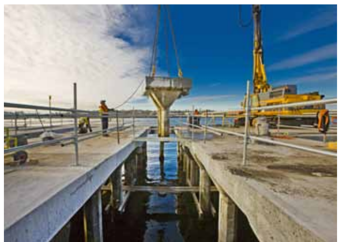
Berth 10 reconstruction adds to container trade capacity.
