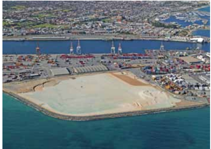
Newly reclaimed land at Rous Head will be used for port-related purposes.
