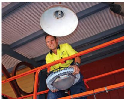
*Installation of energy efficient LED lighting at E Shed.*
