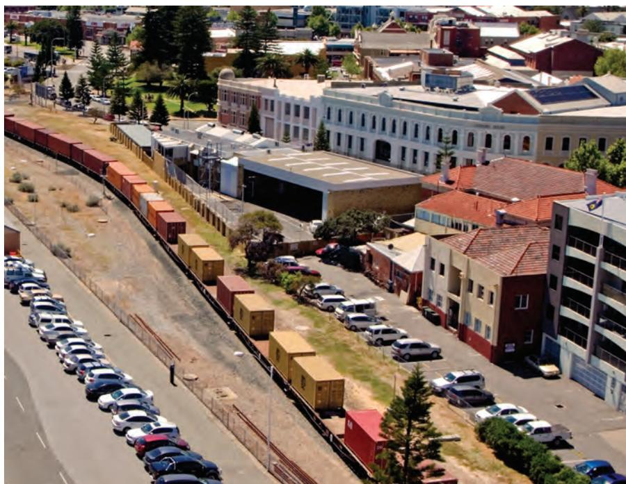
*The rail freight link, which has dual gauge for interstate and intrastate cargo, is vitally important infrastructure for Fremantle Ports.*
