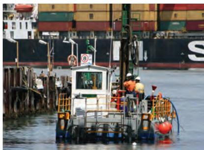
*Core sampling for geotechnical analysis at the Fremantle Rail Bridge.*
