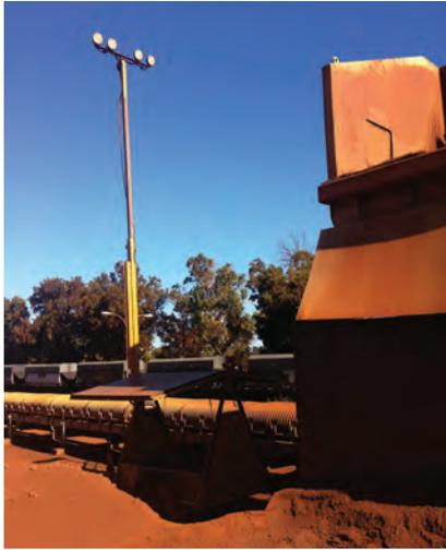
Solar powered lighting tower installed at Kwinana Bulk Terminal.
