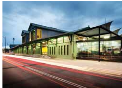
The restored B Shed is a good example of the standard required for C and D Sheds, Victoria Quay Fremantle.
