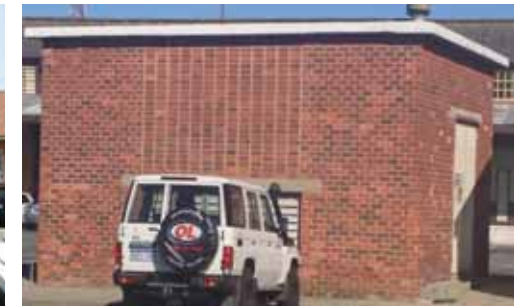
Electrical Substation, Victoria Quay.
