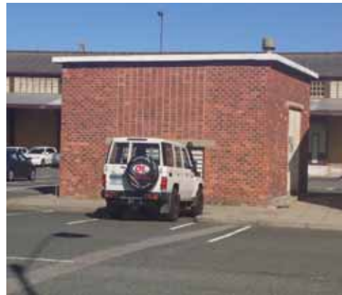
Electrical substation, Victoria Quay.
