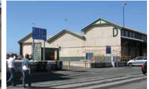
D Shed, Victoria Quay.
