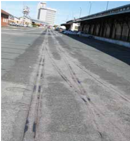
Railway tracks between C Shed and the Old Police Station, Victoria Quay.
