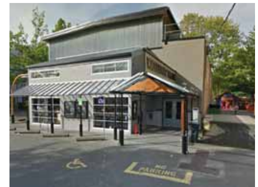
Mechanical equipment discreetly located, Granville Island, Vancouver.
