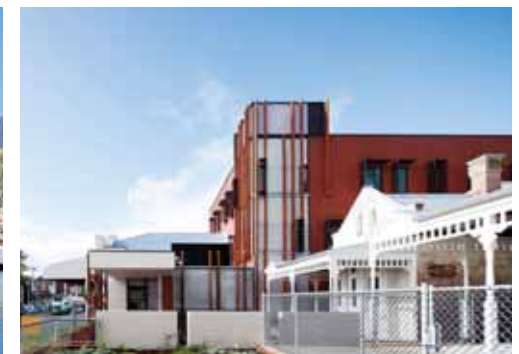
Women's Health Services (WHS) building, Northbridge.
