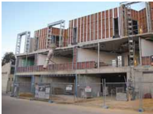
Composite building with reverse brick veneer for the west facing facade, Cottesloe.
