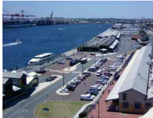
View from E Shed looking across waterfront.
