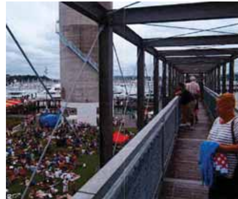
Example of "hi-line", North Wharf Promenade, Wynyard Point, Auckland New Zealand. Taylor Cullity Lethlean Wright + Associates.
