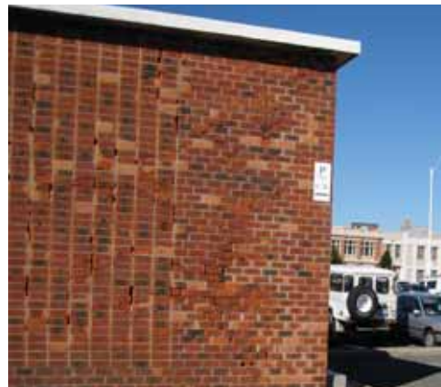
The electrical substation is in poor condition but has an interesting brick layout design.
