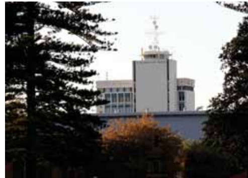
View of Fremantle Ports Administration Building from Esplanade Park, Fremantle.
