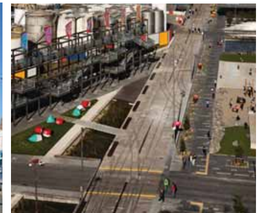
Jellicoe Wharf, Auckland, with railway tracks integrated within the public realm.
