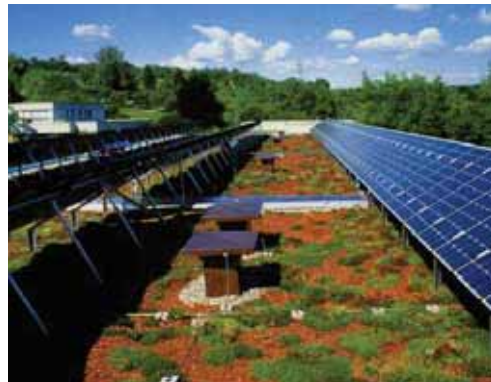
Green roof with solar panels, primary and secondary school, Unterensingen, Germany.
