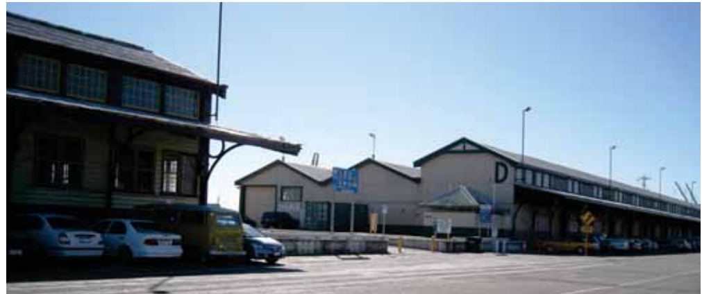
C and D Sheds in the Commercial Precinct, Victoria Quay.
