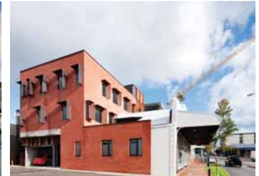
WHS building is a good example of heritage integration required for the Immigration buildings, Victoria Quay.
