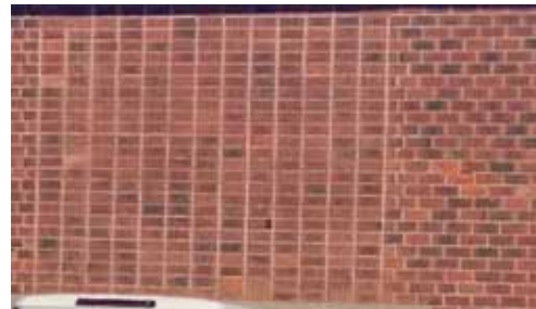
Existing electrical substation brick pattern, Victoria Quay.
