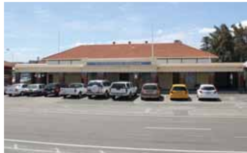
Old Police Station, Victoria Quay.
