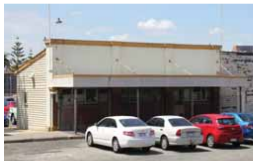
Waiting Room, Victoria Quay.
