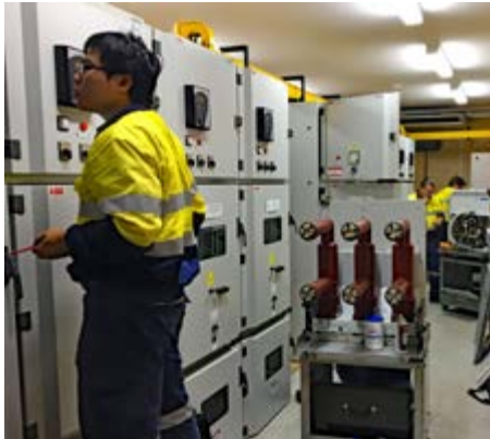
Electrical shutdown checks.
