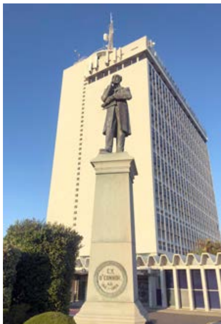
Fremantle Ports Administration Building on Victoria Quay with statue of Fremantle Harbour designer CY O'Connor.
