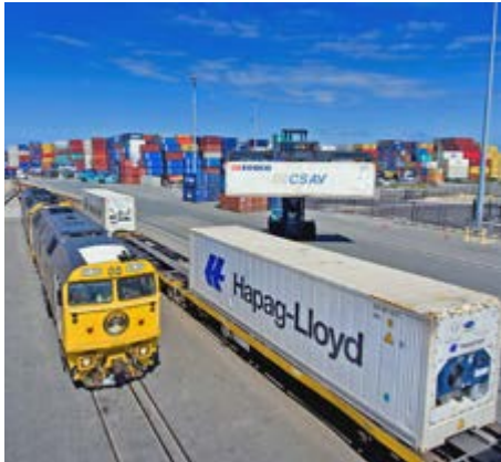
The North Quay Rail Terminal is a modern facility efficiently servicing Fremantle Ports' container trade.
