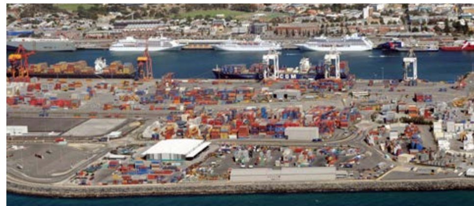
View to Patrick and DP World container terminals, North Quay.
