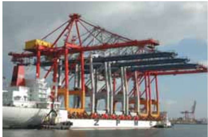
The new $9m post-Panamax container crane was delivered on the Zhen Hua 11, which was carrying five other cranes for other destinations in Australia and New Zealand. The discharge operation took four days to complete.
