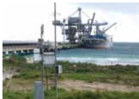
'Real-time dust monitor at the Kwinana Bulk Terminal.
