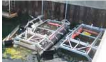
Fremantle Ports has installed a litter trap at Berth 12 (near the railway bridge) to collect litter floating down the river and from boats travelling through the harbour.
