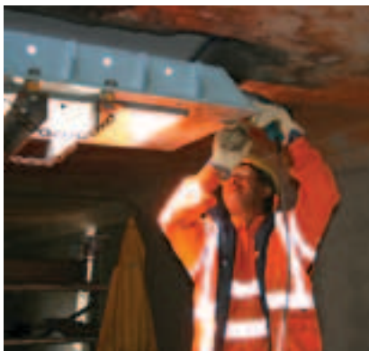
Tunnel repairs at the Kwinana Bulk Terminal.
