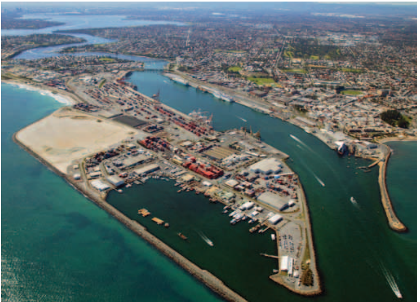
Inner Harbour and Rous Head industrial area
