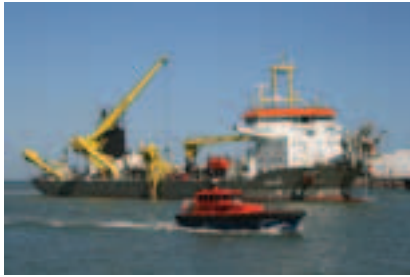
Dredging in the Inner Harbour.
