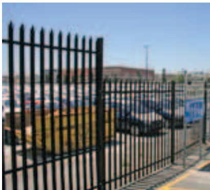
The eastern end of Victoria Quay is a secure zone.
