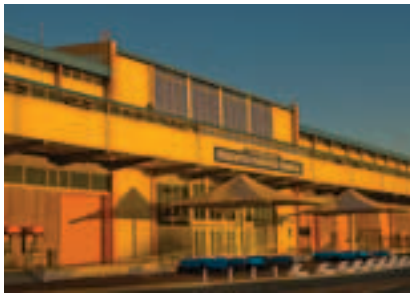
The Fremantle Passenger Terminal, a landmark building on Victoria Quay, was opened in 1960.
