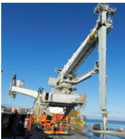
Temporary repairs enabled the Siwertell to go back into service.
