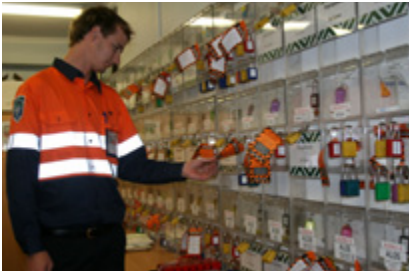
The lockout box system is part of ensuring safe isolation of electrical and other plant.
