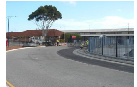
Peter Hughes Drive was realigned for efficiency and safety
