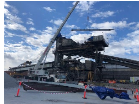
Replacement of the import stacker back stay pendent
