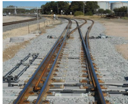
The new 60kg mixed-gauge turnout
