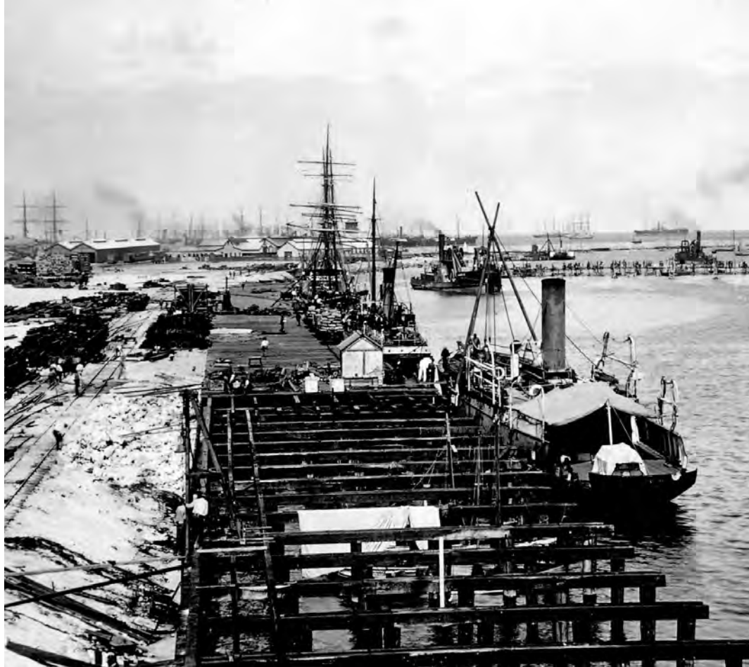
Victoria Quay under construction, 1896 (FP Image C1896.jpg)
